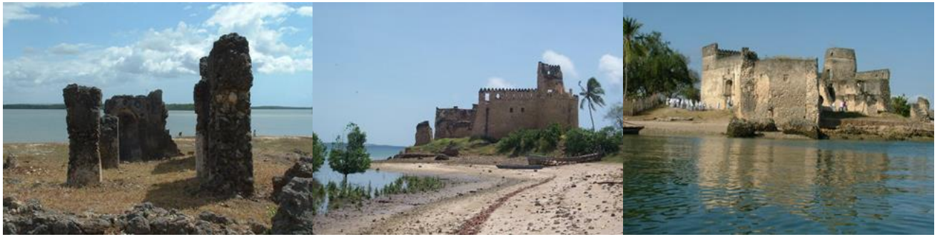
Figure 28: Historical buildings damaged by erosion at Kilwa Kisiwani. Left: location 1. Center and Right: location 2.
