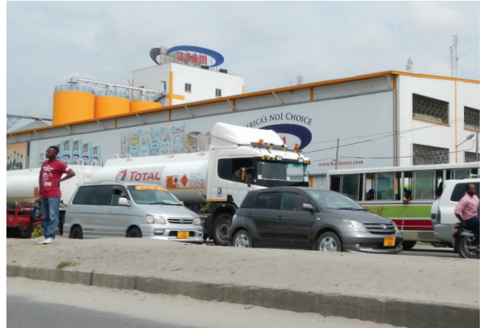
Part of the industrial area of Dar es Salaam
