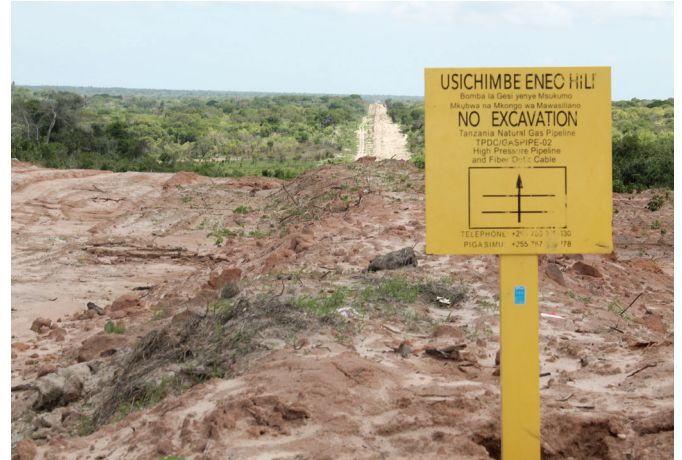
Part of buried gas pipeline in Mtwara, extending to Dar es Salaam
